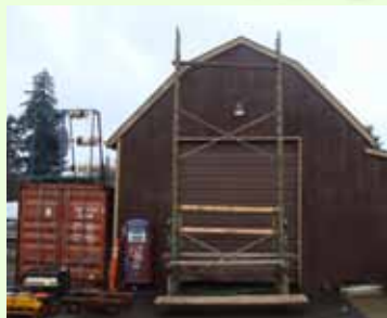
LOTS OF NON-STOP SCAFFOLDING
